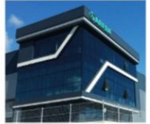
Arfen Bridge and Building Technology Company / İZMİT
