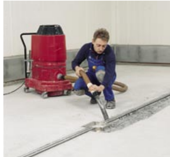
Vacuuming up dust and dirt
