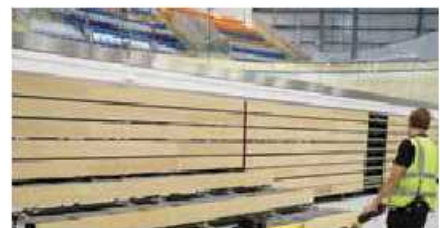
ICC at ExCel London, UK.
