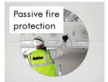
Intumescent Coatings, Fire Stopping
