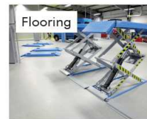
Seamless Resin Flooring, Subfloor Preparation, Car Parking Structures
